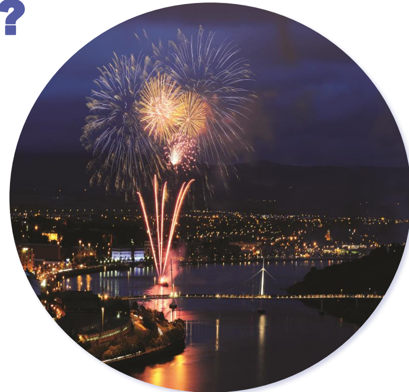
The Peace Bridge Derry-Londonderry
